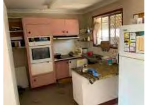
Showing examples of obstructions (e.g. wall, floor, ceiling coverings, cabinets, window furnishings, vegetation, insulation and ducted AC, furniture and stored goods, etc.)
