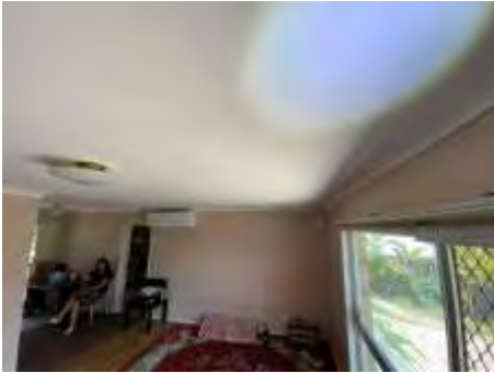
Showing examples of obstructions (e.g. wall, floor, ceiling coverings, cabinets, window furnishings, vegetation, insulation and ducted AC, furniture and stored goods, etc.)
