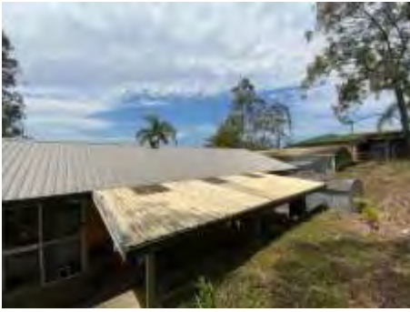
Showing example of upper roof
