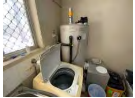
Showing examples of obstructions (e.g. wall, floor, ceiling coverings, cabinets, window furnishings, vegetation, insulation and ducted AC, furniture and stored goods, etc.)
