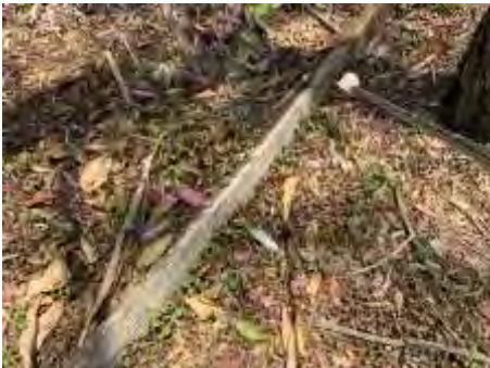
Wood rot to parts of the retaining walls. Recommend engaging a builder to repair/replace and avoid further deterioration
