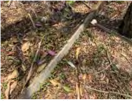
Showing example of fungal decay to timber
