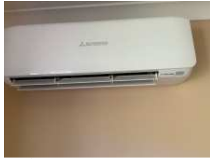
All AC units were working at the time of the inspection, but for a proper testing and gas measurement, a AC technician needs to be engaged
