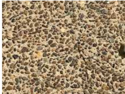
Settlement cracks to parts of the pathway/driveway. Recommend engaging a concreting contractor to repair/replace and avoid further deterioration
