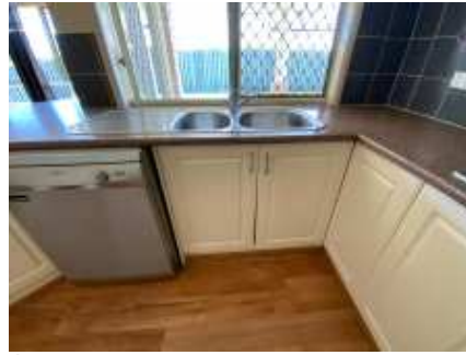
Showing cabinet door needs adjustment
