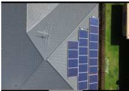
Showing the solar panel on top of the roof
