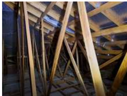
Showing example of roof space
