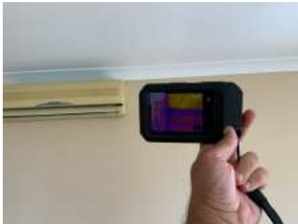
The property shows signs of termite damage. Due to the possibility of concealed structural damage recommend removing any linings that may be concealing structural damage and properly assessing the structural integrity of the building. Recommend engaging a builder to undertake an invasive building inspection and undertake any repairs necessary. Recommend the above be implemented as soon as practical
