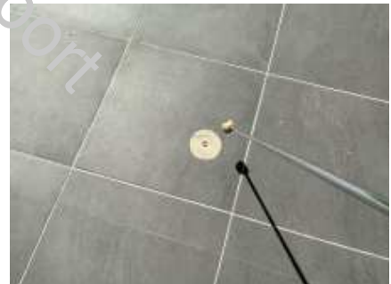
Showing bait station installed around the house.
