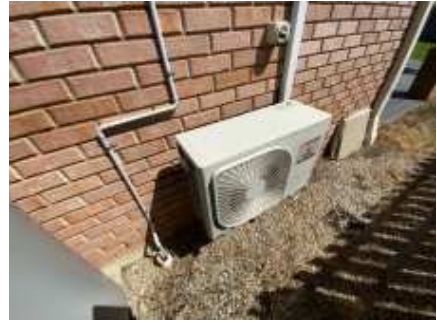
Showing example of the bridging/breaching
