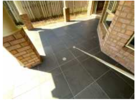
Showing bait station installed around the house.
